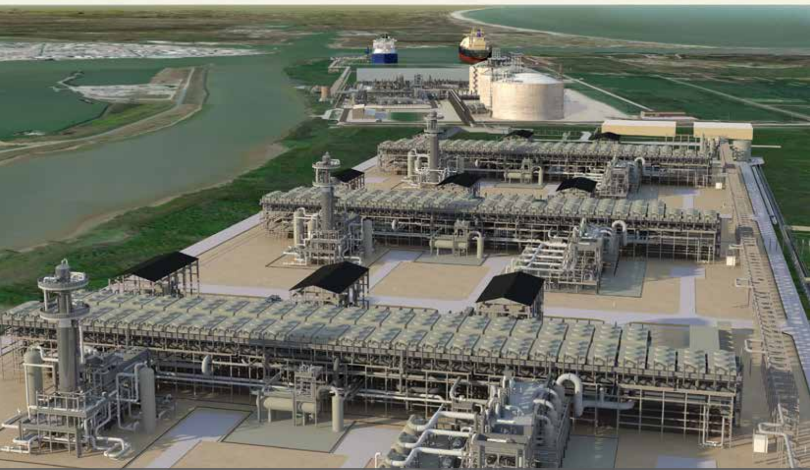
Freeport LNG's liquefaction construction, shown as a model, could be hindered by election year politics.
