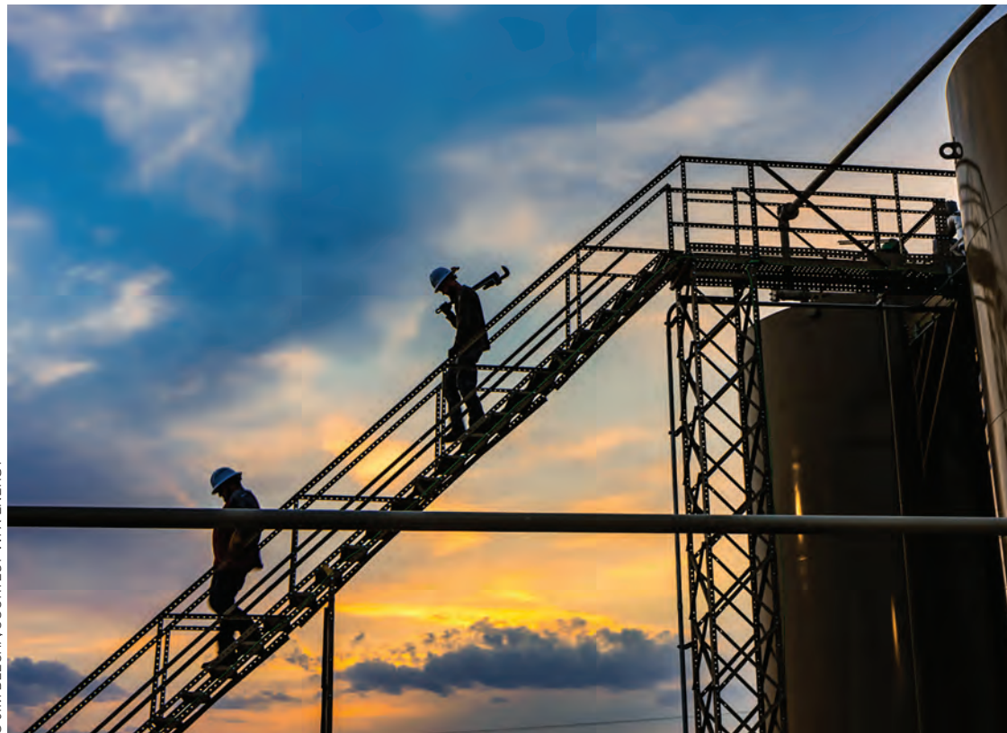
WPX workers at the Lindsay Compressor Station.
