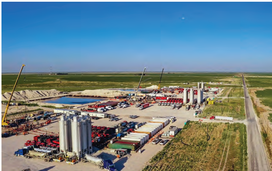
Solaris Oilfield Infrastructure Inc. silos of proppant at a multilwell pad in the Permian Basin.
