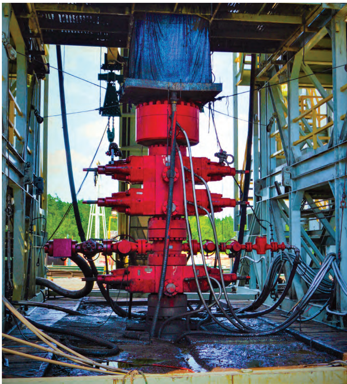
A blowout preventer at Camino’s Cora Mae 10-15-1H well, which is located in Grady County, Okla. Parent/child interactions pose challenges in the areas where Camino operates.
