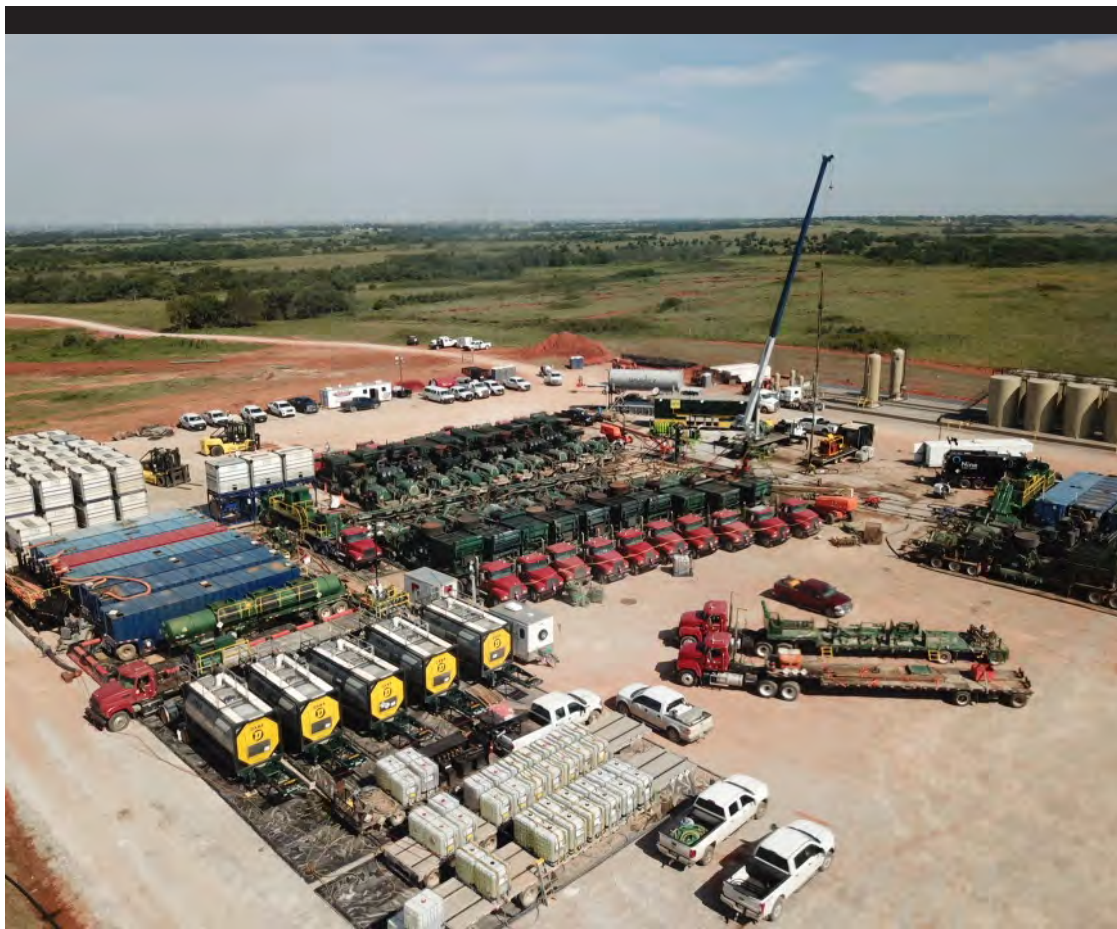
A hydraulic fracturing spread is on location at a Camino well site in Grady County, Okla.
