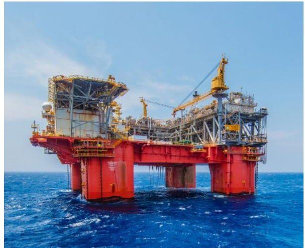
The Atlantis Phase 3 project will include constructing a new subsea production system from eight new wells that will be tied to the existing platform. (Source: BP)
