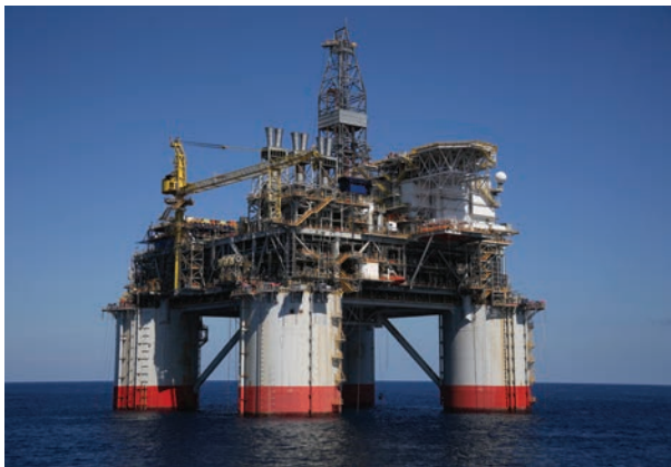
The Chevron-operated Big Foot project uses a 15-slot drilling and production tension-leg platform, the deepest of its kind in the world. (Source: Business Wire)
