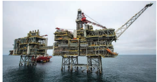
The Clair Ridge Field is the site of the first offshore deployment of BP's LoSal EOR technology. (Source: BP)
