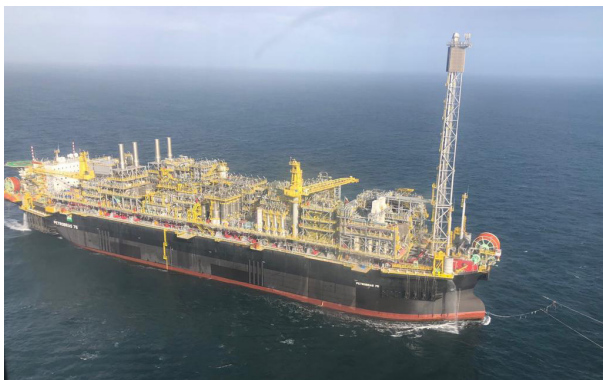
The platform is Petrobras’ fourth to start production in 2018. (Source: Petrobras)
