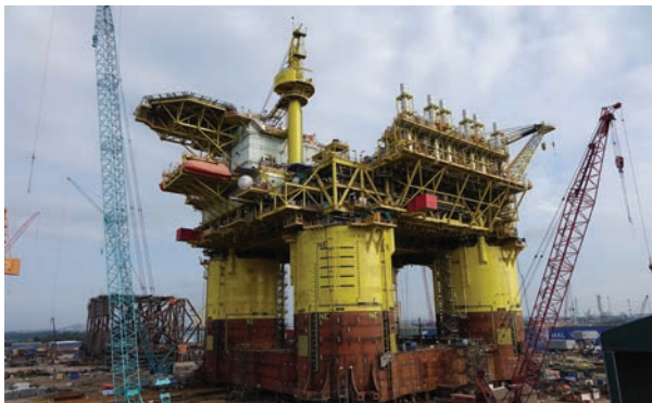
Shell's deepwater Malikai TLP, destined for offshore Malaysia, is the company's first such platform designed and built outside the Gulf of Mexico. (Photo courtesy of Shell)
