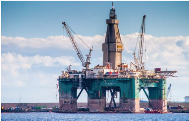
The contract for the Eirik Raude has been terminated.
