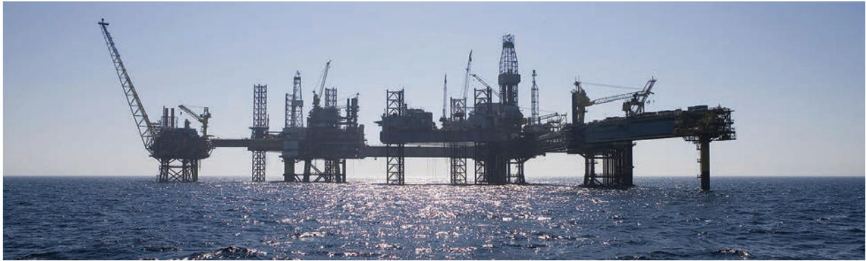
The Dan Field has undergone subsea lifetime extension work.
