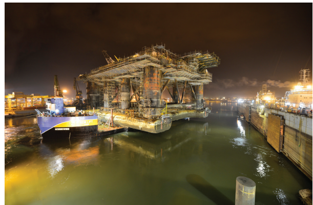
Work on the FPF-1 is taking longer than expected.
