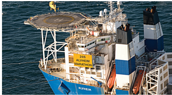
Bøyla is tied back to the Alvheim FPSO.
