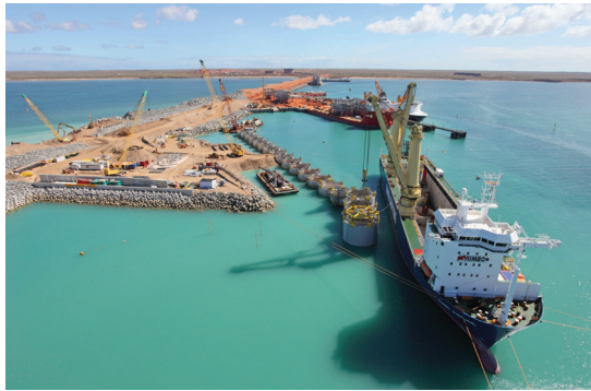
Gorgon is now in final stages of commissioning.
