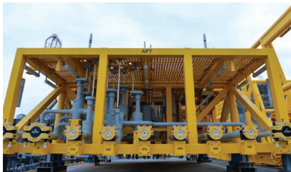
The Gullfaks compressors have been removed from the seabed.
