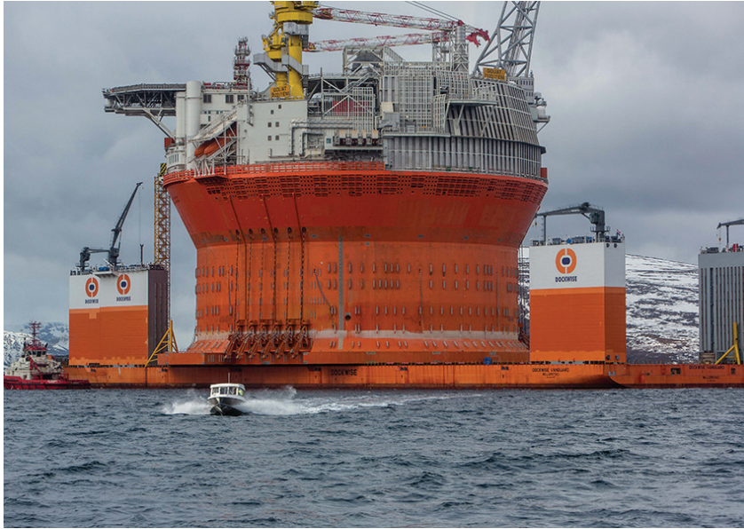
The subsea power link to Goliat has been commissioned.
