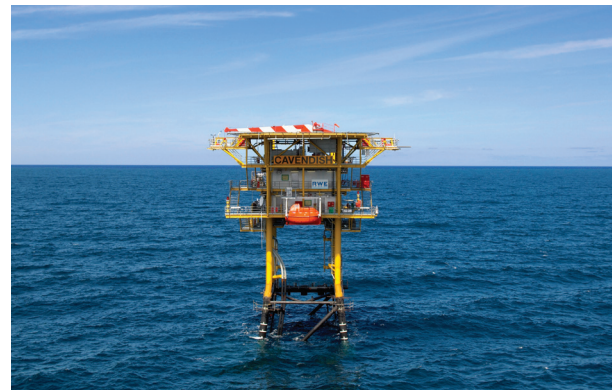
The unmanned Cavendish platform in the UK North Sea.
