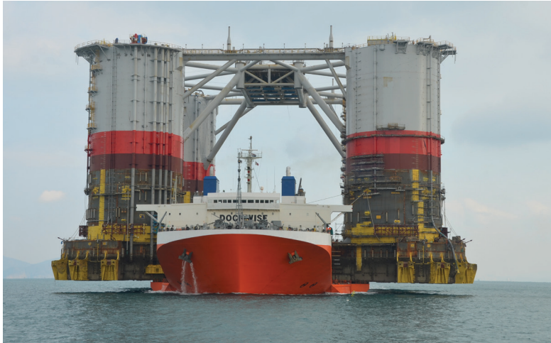
Big Foot has returned to Kiewit's Ingleside, Texas, yard.
