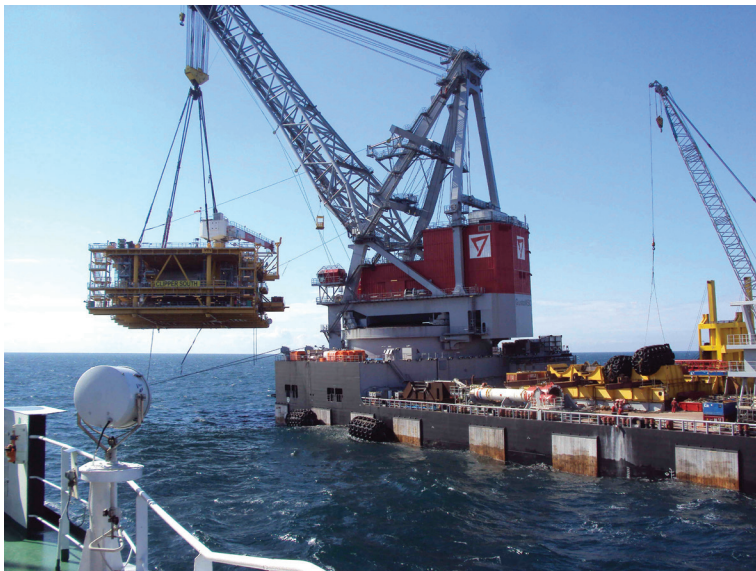
The Clipper South topsides being installed.
