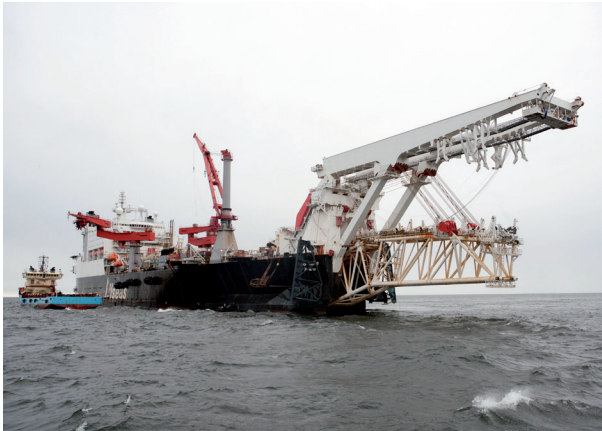
The Solitaire has completed laying the Polarled pipeline.
