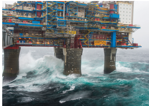
Alfa Central will be tied back to Sleipner infrastructure.
