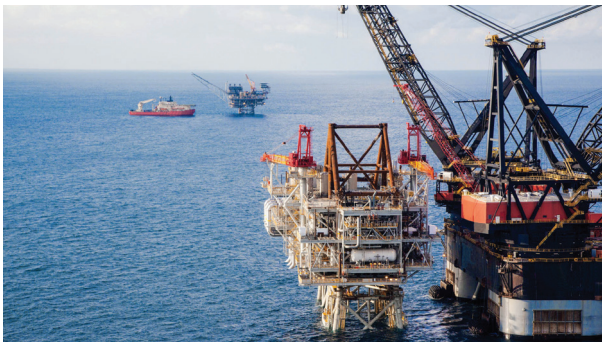
Infrastructure being installed on the Tamar field.
