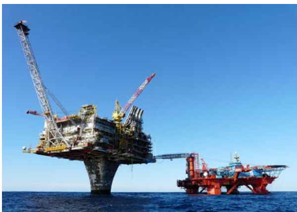
Shell's Draugen platform
