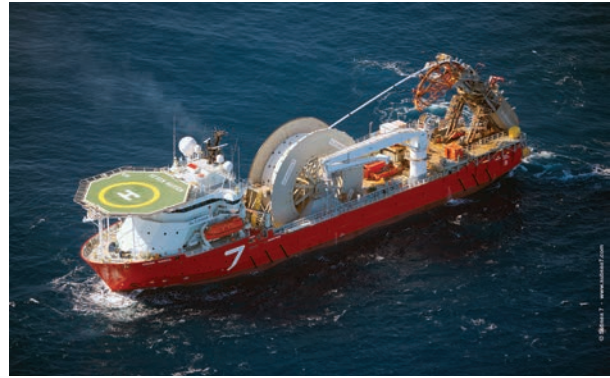
The Seven Navica is installing pipelines on Mariner
