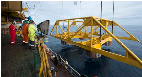
The Åsgard template being installed
