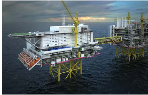
The Johan Sverdrup utility and living quarters platform
