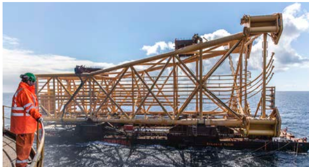
The Ivar Aasen jacket being installed
