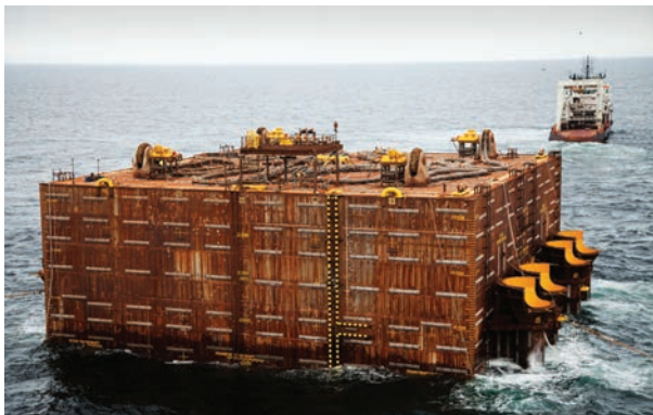
Oil is stored in the Solan Field's subsea tank.
