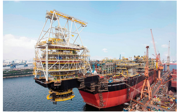
The Tullow Oil-operated TEN Field development, located offshore Ghana, utilizes an FPSO. (Source: Tullow Oil)
