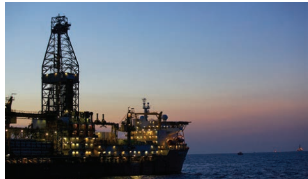
An FPSO operates offshore Mozambique where Anadarko Petroleum and partners are working to develop fields in Offshore Area 1. (Source: Anadarko)
