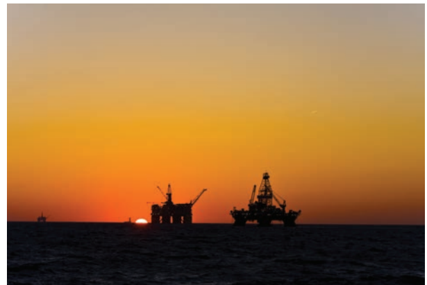
Oil platforms are positioned in the U.S. Gulf of Mexico. The U.S. government is gearing up for a lease sale in March. (Source: Shutterstock.com)
