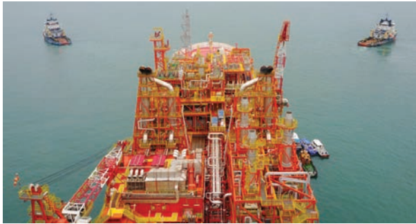
EnQuest continues to bring down costs at the Kraken oil field in the North Sea. (Source: EnQuest)
