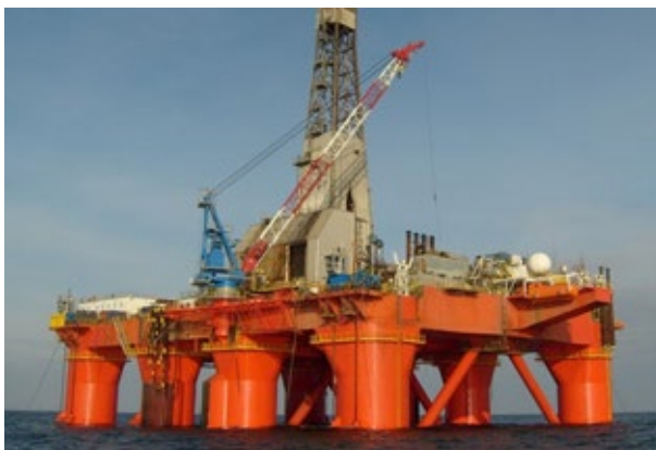
Both wells were drilled by the Paul B Loyd Junior rig in summer 2017. (Source: BP)
