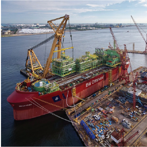
The BW Catcher FPSO vessel is used to produce oil from the Catcher Field in the North Sea. (Source: BW Offshore)
