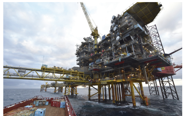
The redevelopment plan includes a new processing platform and a new accommodation platform for Tyra East (shown here) and Tyra West. (Source: Maersk Oil)
