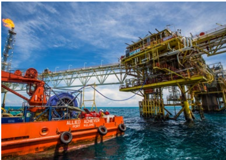
The IFL technology was recently installed offshore Malaysia. (Source: APS)
