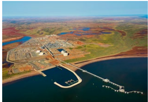
Chevron has achieved first LNG production at Wheatstone. (Source: Chevron)
