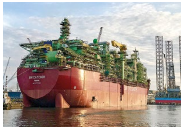
The Catcher FPSO unit is undergoing a conversion to use in the North Sea in the Keppel Shipyard in Singapore. (Source: Premier Oil)
