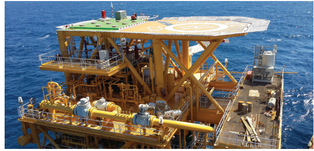
The Sea Swift was installed in 23 m water depth and from design to installation took 18 months to complete. (Source: Aquaterra Energy)
