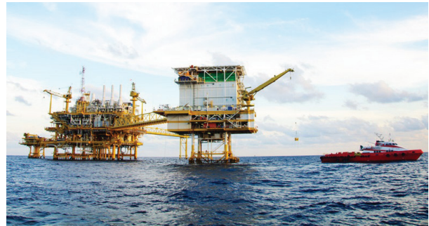
The Marjan oil field is located off Saudi Arabia's east coast. (Source: Amec Foster Wheeler)
