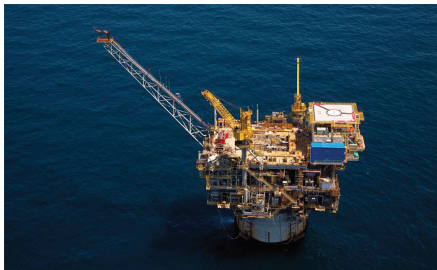
Anadarko's 100%-owned Constitution spar in the Green Canyon area of the deepwater U.S. GoM will host production from the Constellation Field roughly 32 km (20 miles) away.
