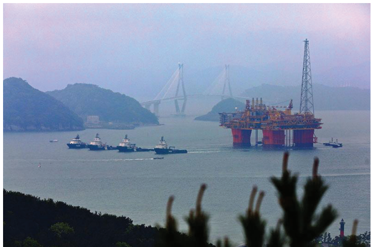
The INPEX-operated Ichthys LNG Project's CPF sailed away from its construction site in Geoje, South Korea, en route to the Ichthys Field offshore Western Australia. (Source: Inpex)
