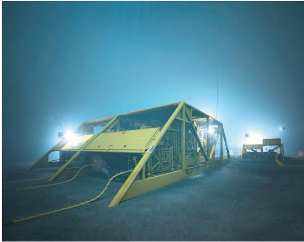
Both trains for the Åsgard subsea compression system are installed on the seabed. (Source: Aker Solutions)
