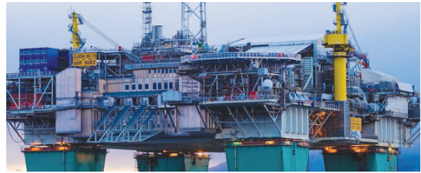
The Gjøa platform is a semisubmersible production unit that has full processing and export capabilities. (Source: Engie)
