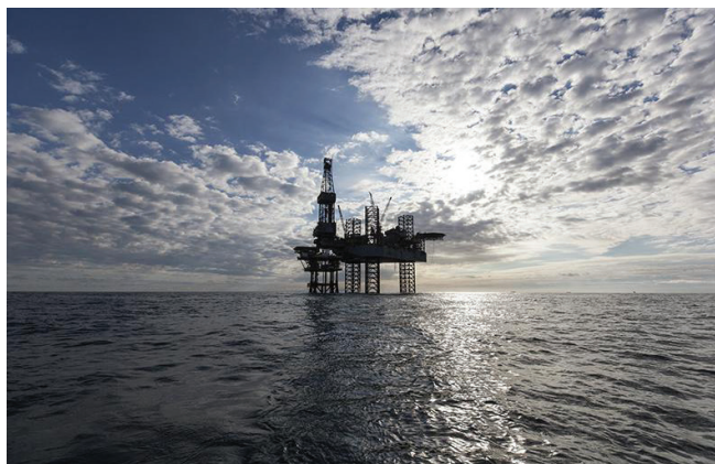
At 200, subsea tieback opportunities lead the development options for marginal fields in the U.K. North Sea.
