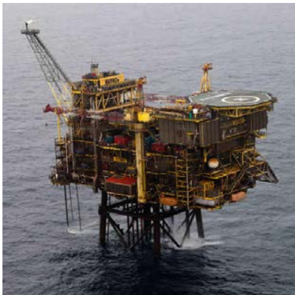
Subsea wells at the Scolty/Crathes development will be tied to the Kittiwake platform. (Source: Centrica)
