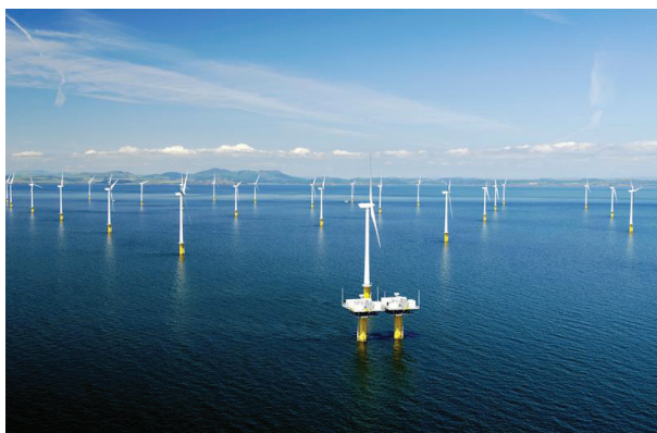
Offshore wind turbines generate energy at the Robin Rigg wind farm off the coast of Dumfries, Scotland. (Source: Scottish Enterprise)
