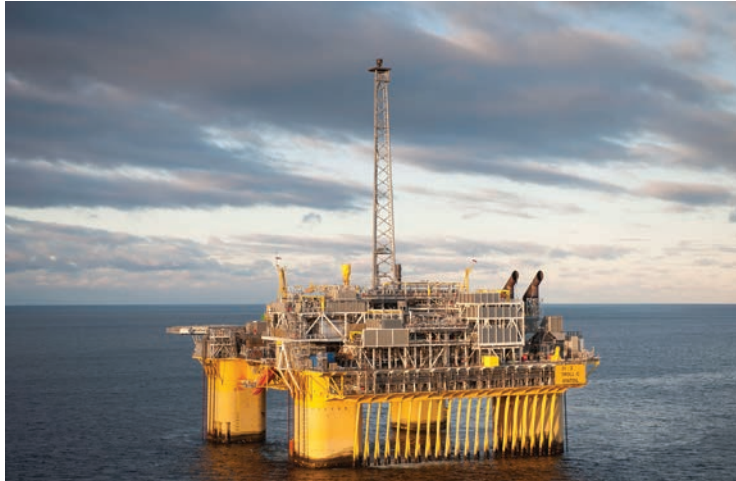
Production from Fram C East will be tied back to the Troll C platform hub. (Source: Øyvind Hagen /Statoil ASA)
