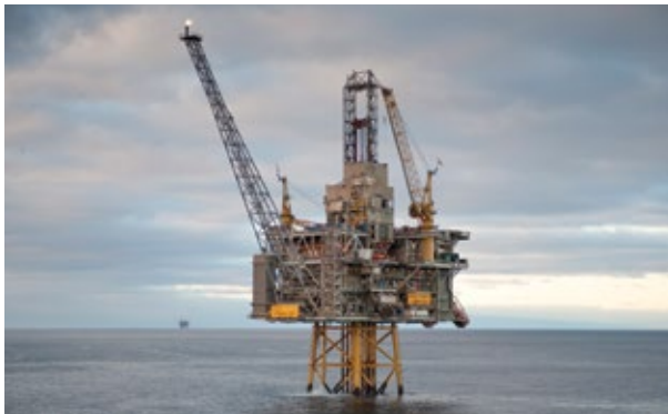
The Oseberg Ost platform off Norway
