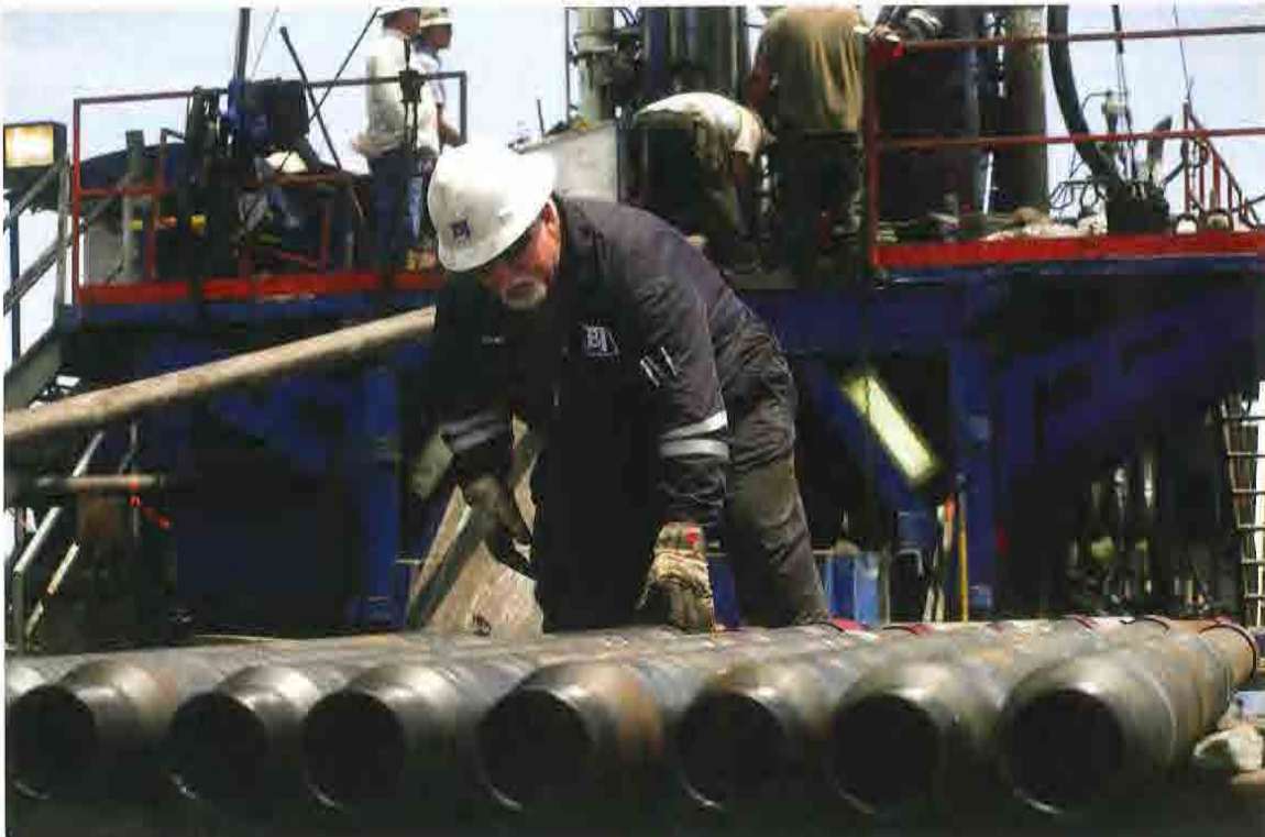
The DirectStim multistage completion system provides an efficient means to ensure proper treatment volumes reach the entire length of long, open-hole horizontal wells in the Permian Basin. (Photo courtesy of BJ Services)
