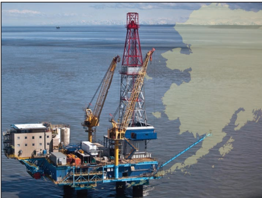
Miller Energy's Osprey Platform is part of its Cook Inlet midstream infrastructure.
