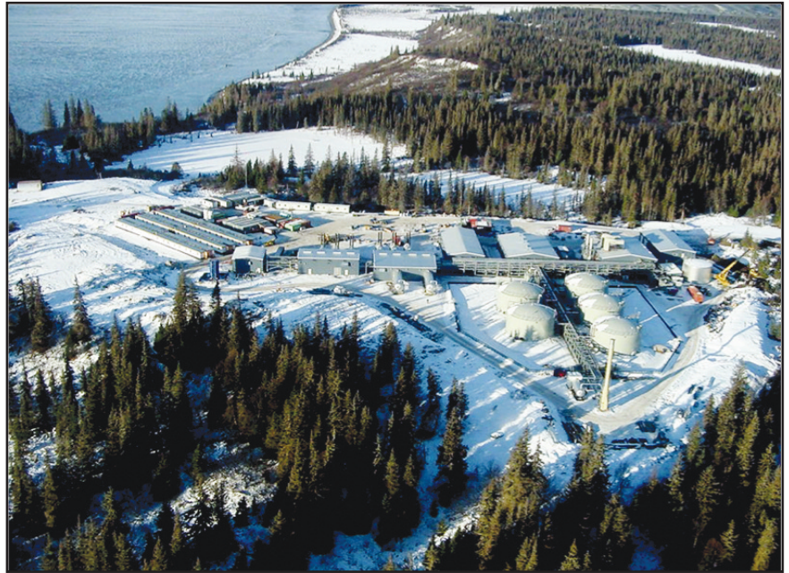
The Kustatan Production Facility in Alaska is a state-of-the-art midstream asset that Miller Energy purchased.
