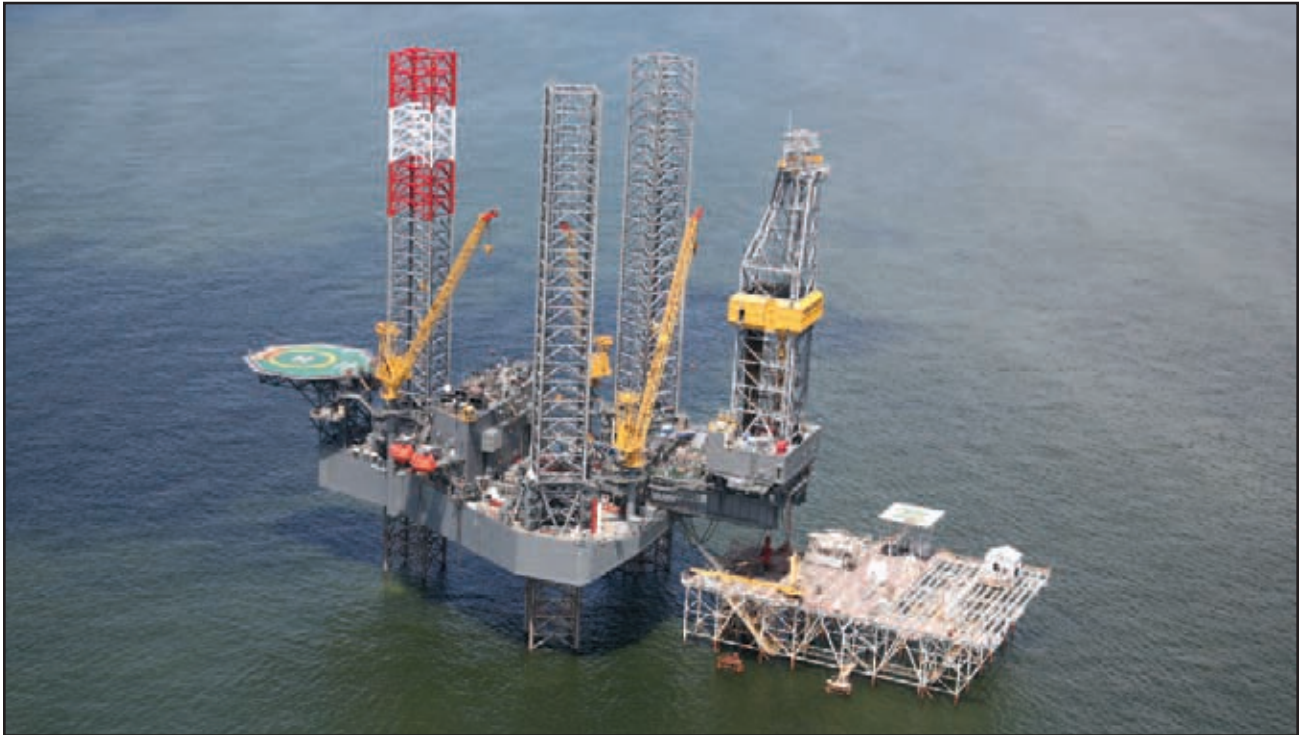
The Rowan EXL III drilling rig at the Grand Isle field in 2011.
