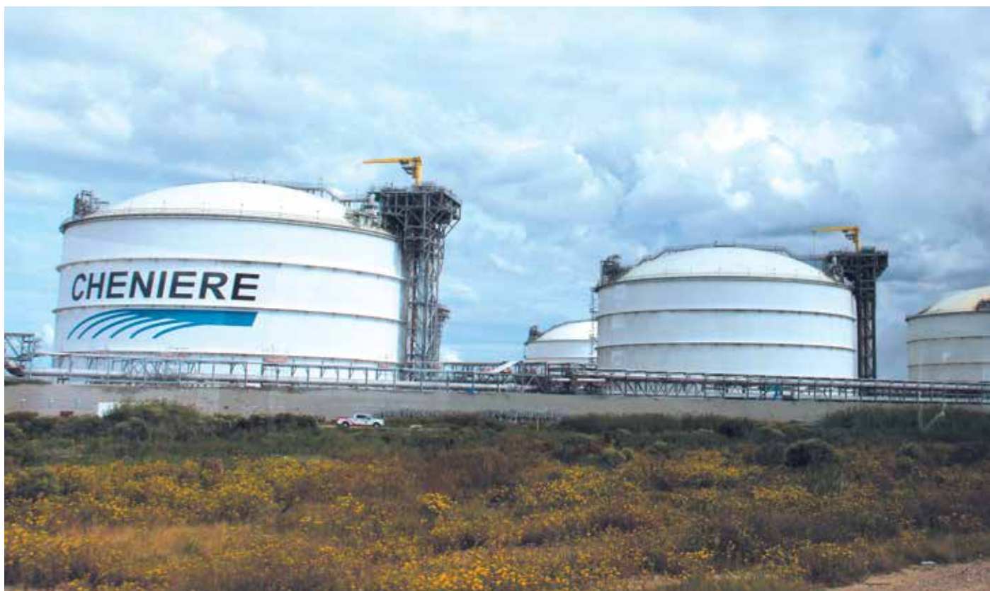
Cheniere Energy’s Sabine Pass plant in Louisiana put the U.S. on the map as a major LNG supplier. The rapidly expanding gas export business has helped the firm emerge as one of the midstream sector’s biggest players. Source: Cheniere Energy Inc.
