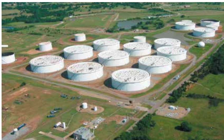
You can’t beat midstream infrastructure like this—Oklahoma’s sprawling Cushing pipeline, storage and trading hub. This is Blueknight Energy’s share of the complex with nearly 6.6 million barrels of storage. In all, Blueknight operates 7.8 million barrels of storage for Midcontinent producers.
