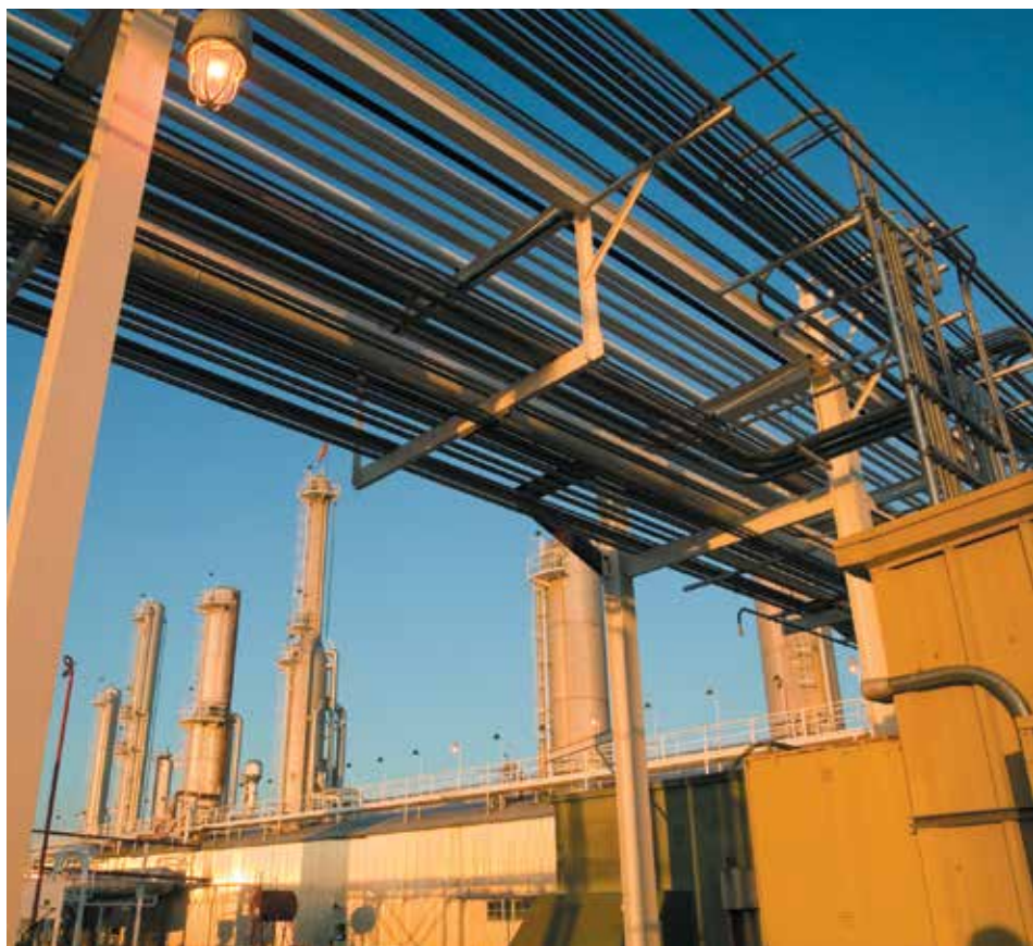
The Opal, Wyo., gas processing plant of The Williams Cos. Inc. has emerged as a natural gas pipeline and storage hub for much of the Intermountain West. Source: The Williams Cos. Inc.
