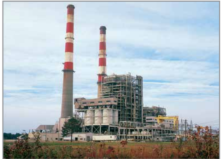
Out To Pasture | Duke Energy's coal-fired Sutton plant (above) is being retired after 59 years of service as the company began operating a new 625 MW combined-cycle gas-fired plant. (Courtesy: Duke Energy)
