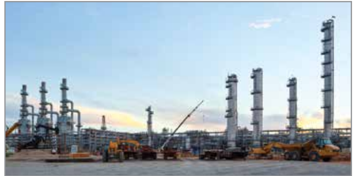
Growing | ONEOK Partners’s MB-2 fractionator will supplement the company’s 160,000 bbl. per day MB-1 fractionator by adding 75,000 bbl. per day of capacity at Mont Belvieu. (Courtesy: ONEOK Partners LP)
