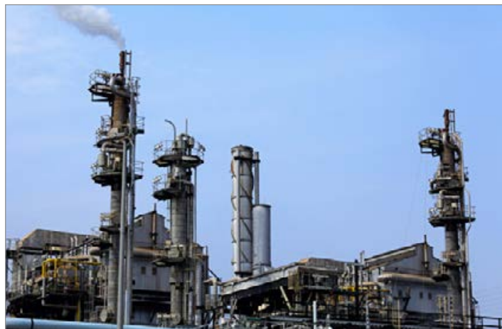
ADDING INFRASTRUCTURE | Eagle Rock completed a $227.5 million deal for BP America's two processing plants and gathering system in the Texas Panhandle.
