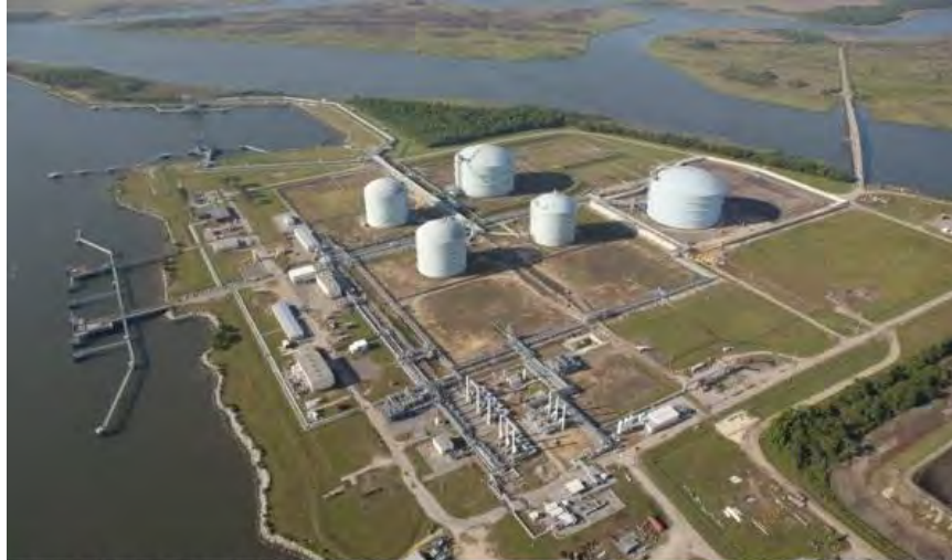
Pictured is the site of the proposed Elba Liquefaction Project at Elba Island Terminal near Savannah, Ga. (Source: Kinder Morgan Inc.)
