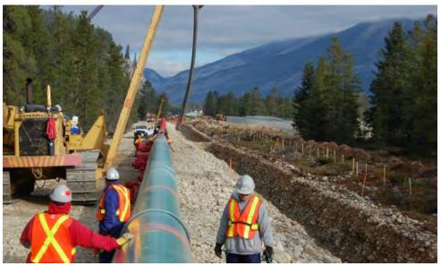
A crew positions pipe for the Anchor Loop section of Kinder Morgan Inc.'s Trans Mountain Pipeline expansion. Completion of the system has been delayed by opposition from an environmental movement determined to stop the company from acquiring the necessary permits, Chairman and CEO Rich Kinder told industry executives at the recent IHS CERAWeek conference in Houston. Source: Kinder Morgan Canada Inc.
