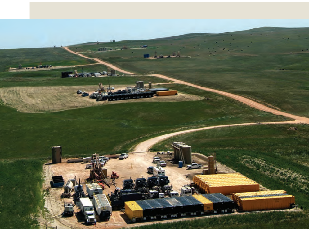
Results from simultaneous fracture stimulations on three wells in Montana demonstrate the potential benefits of these enormous operations, but the logistics are daunting. (Photo courtesy of BJ Services Co.)
